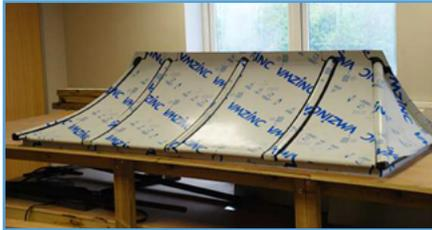
If a protective layer is fitted to the canopy, this must be removed **after** installation. If the protective film gets wet this may cause staining to the covering.
