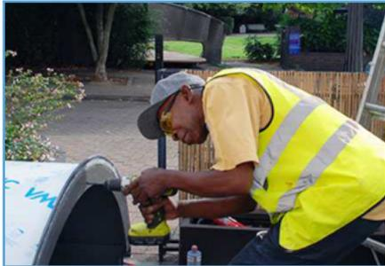
All of the Zinc & Copper canopy frames and brackets will need to be drilled by the installer prior to installation to locate the correct fixing points in the substrate.
