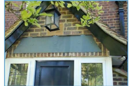
The flashing will need to be cut and chased and pointed with a proprietary sealer by the installer as necessary.
